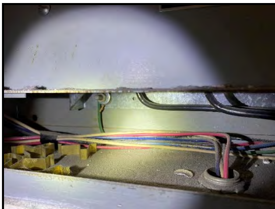
Figure 5 (left): Non-compliant grounding to panel housing
