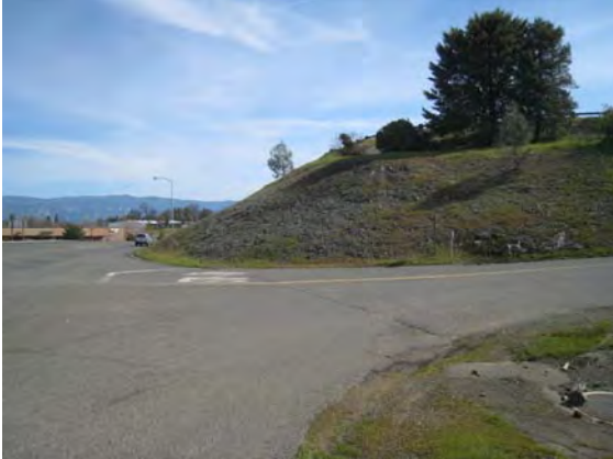
Northbound approach looking east
