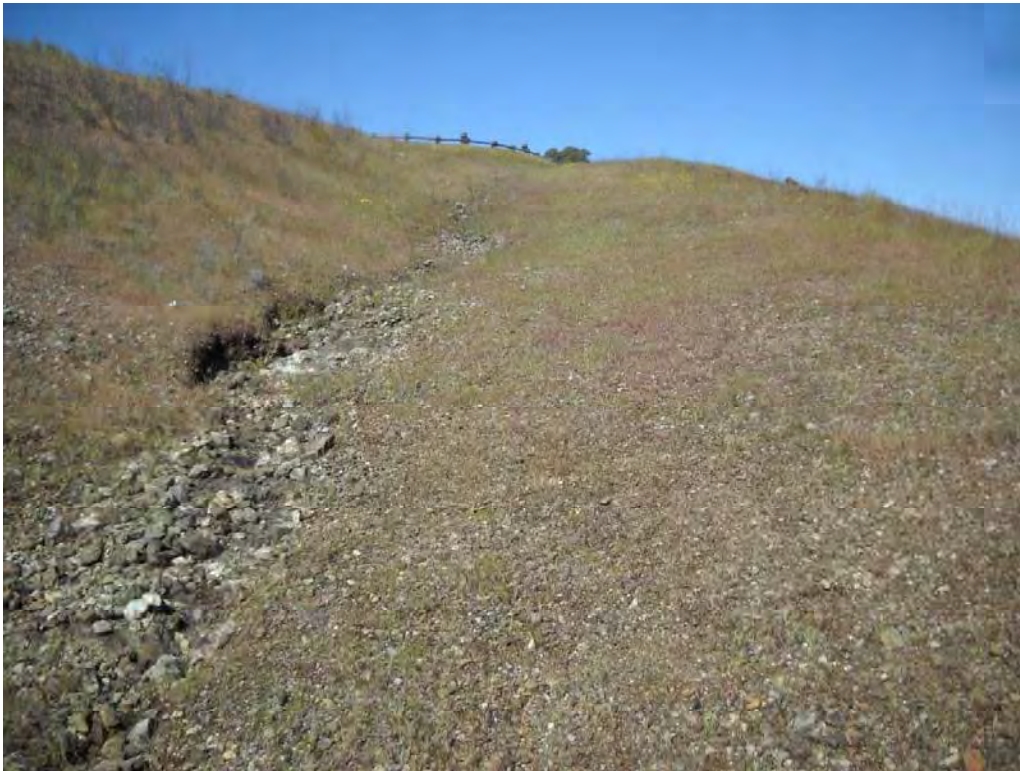
Constructed Drainage Ditch 4/29/10
