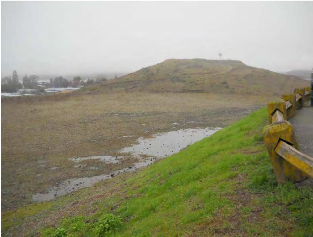
Ponded Water on Upper Terrace 2/8/10
