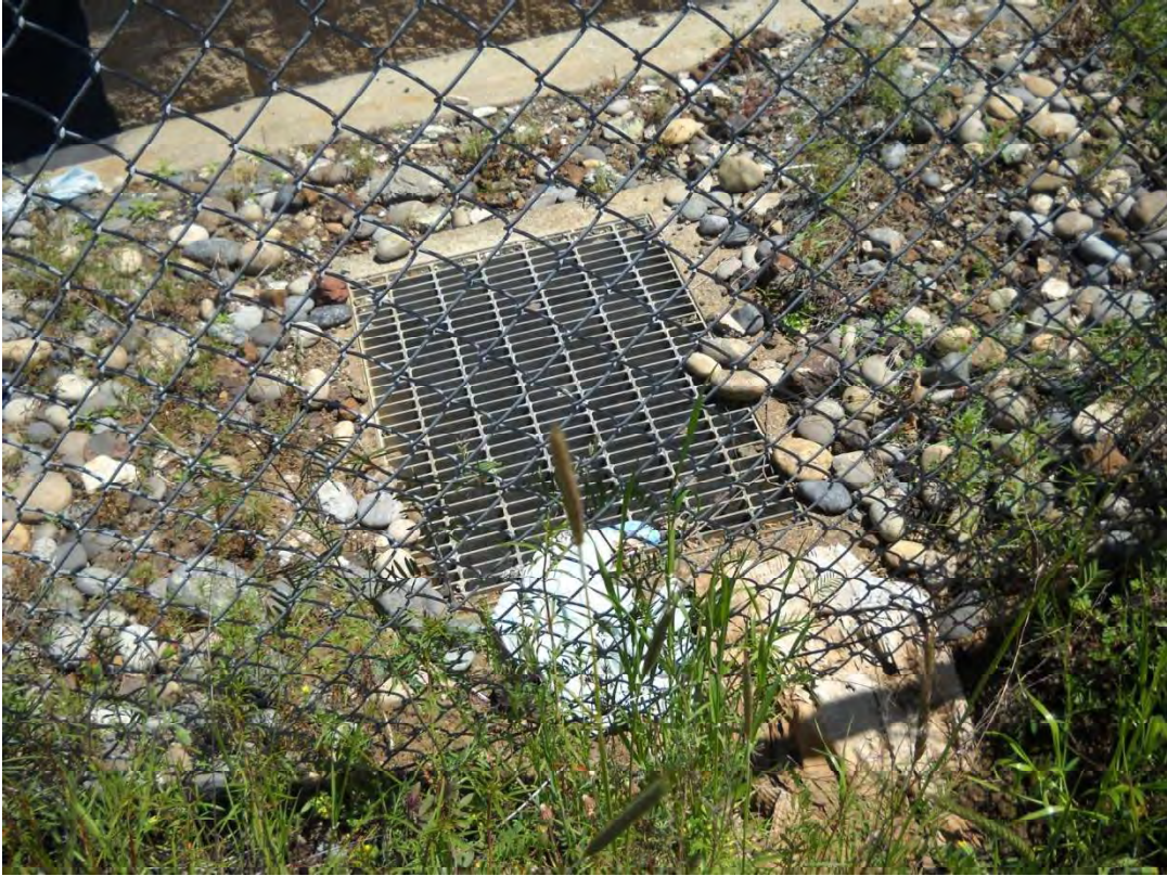
Storm drain inlet at terminus of 8:CD 4/29/10
