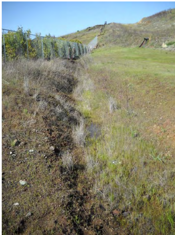
8:CD looking west toward culvert 3/17/10
