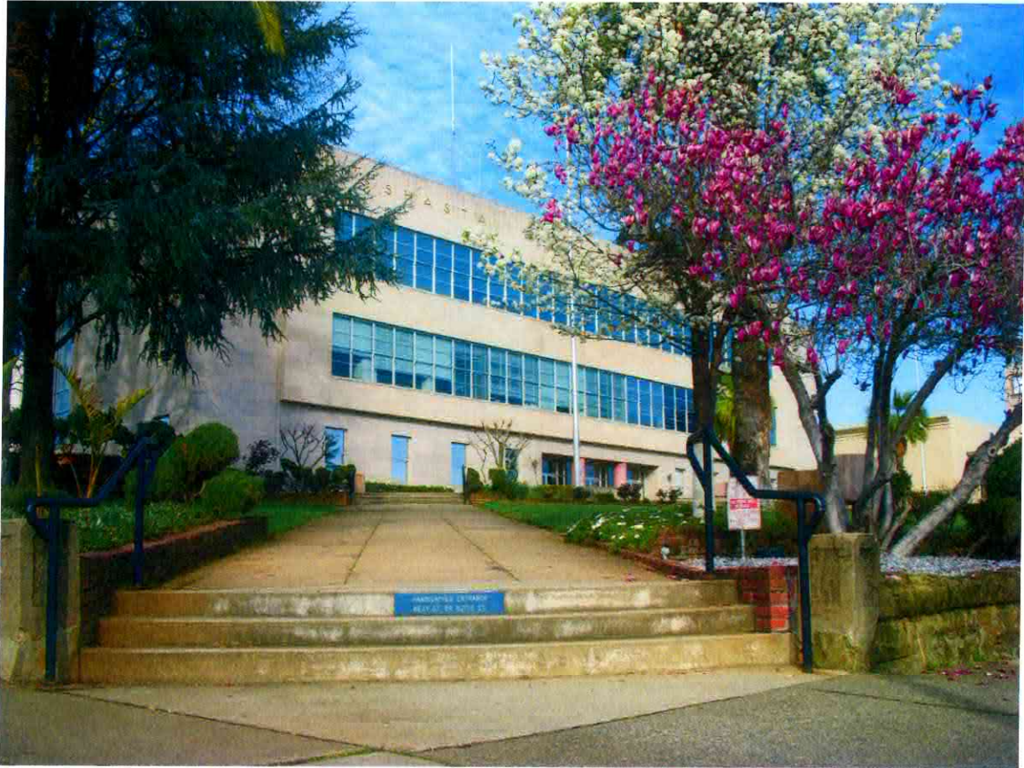
Front of courthouse, steep slope, stairs and ADA access
