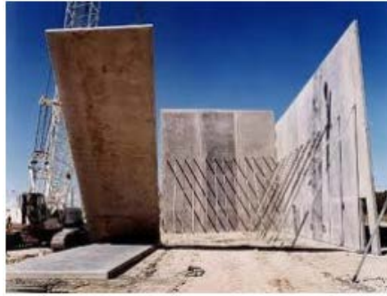
Three images of tilt-up construction in action
