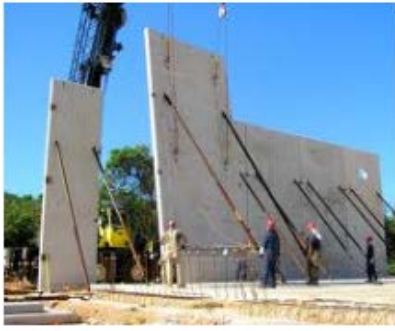
Three images of tilt-up construction in action
