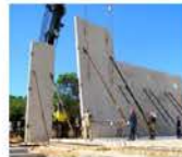
Tilt-Up Concrete Construction
