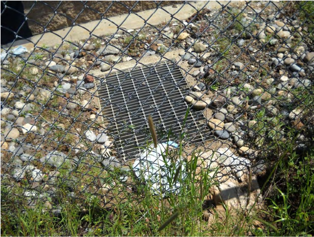
Storm drain inlet at terminus of 8:CD 4/29/10
