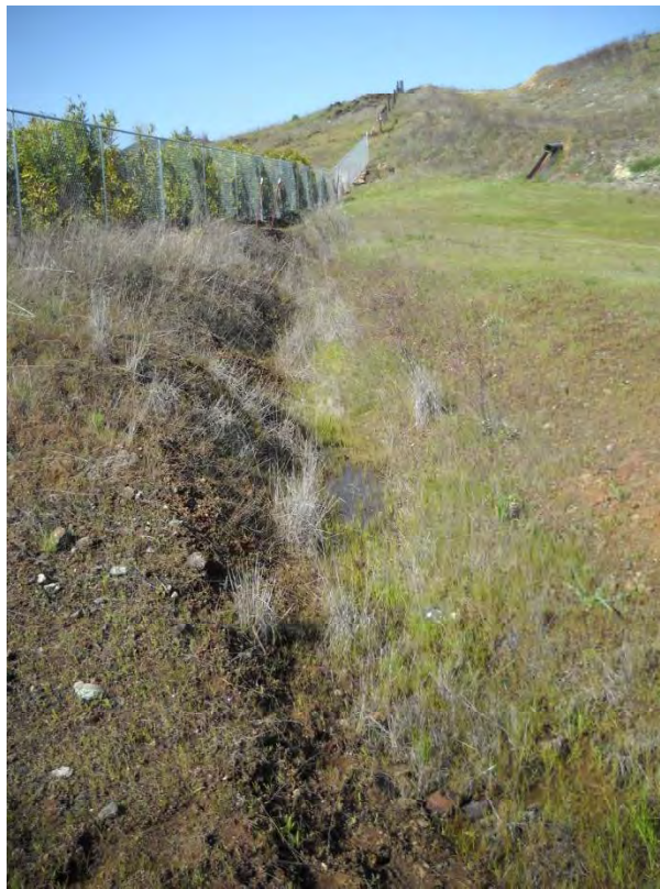
8:CD looking west toward culvert 3/17/10
