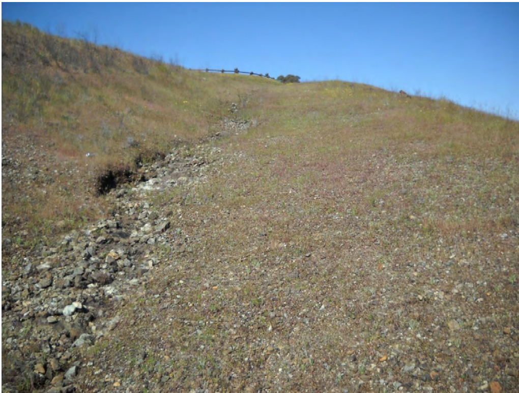
Constructed Drainage Ditch 4/29/10
