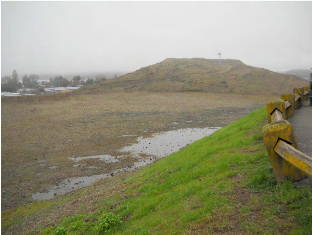
Ponded Water on Upper Terrace 2/8/10
