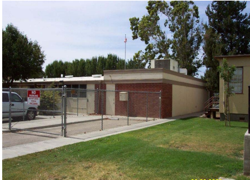
FIGURE 2.7.2a In-custody Defendants Loading/Unloading from Vans in an Unsecured Area
