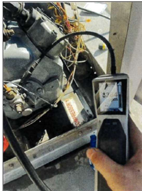
Testing for refrigerant leak
