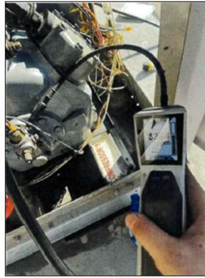
Testing for refrigerant leak
