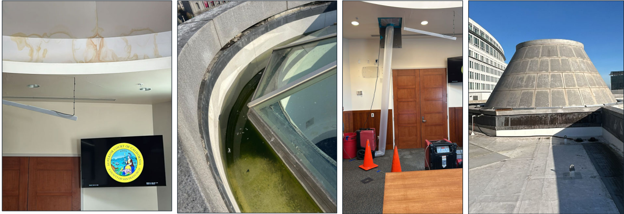
FM-2010629 – Civic Center Courthouse – Roof
