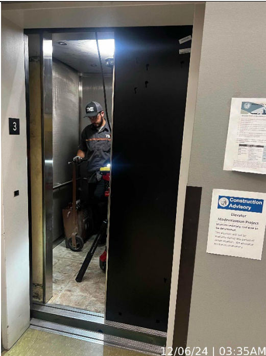
Hayward Hall of Justice - Elevator
