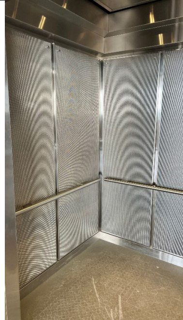
East Los Angeles Courthouse – Elevators
