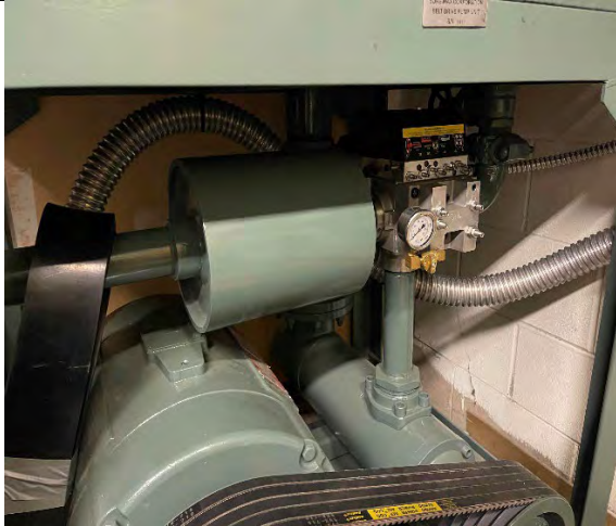
Fremont Hall of Justice - Elevator
