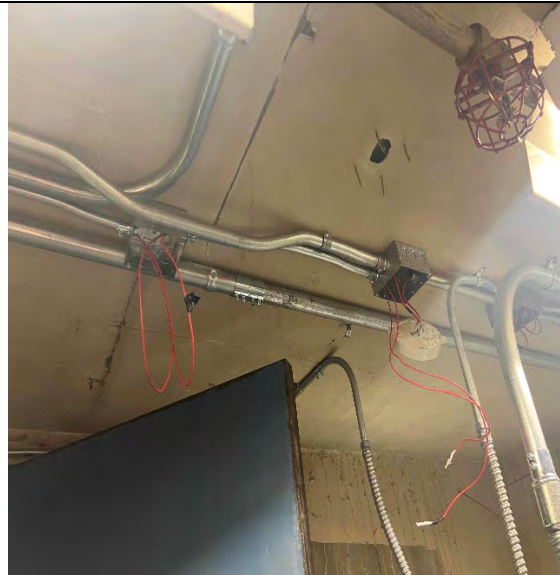
Hayward Hall of Justice - Elevator
