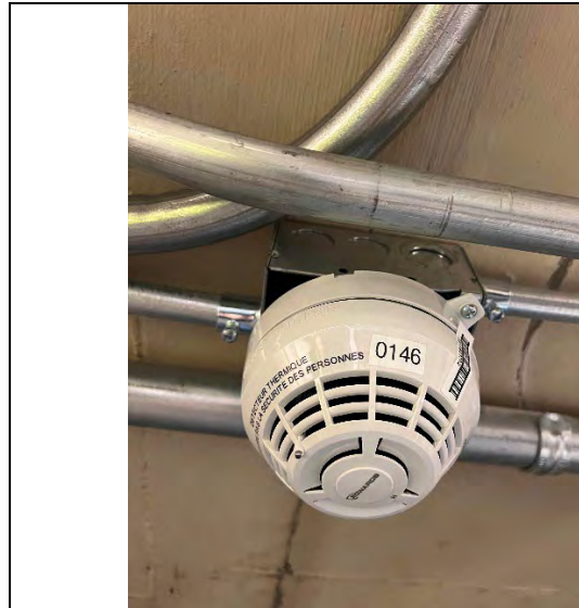
Hayward Hall of Justice - Elevator
