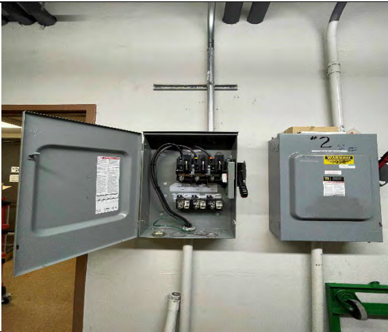
Fremont Hall of Justice - Elevator
