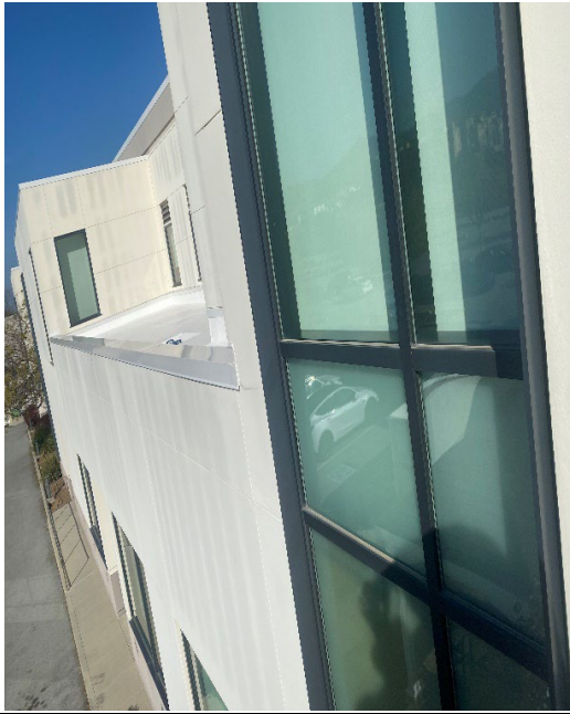
Morgan Hill - Roof
