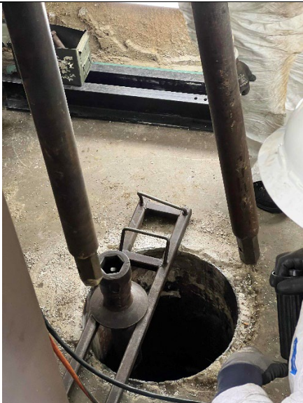
Hayward Hall of Justice - Elevator
