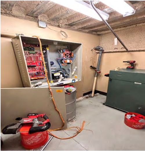
Harbor Justice Center-Newport Beach - Elevators
