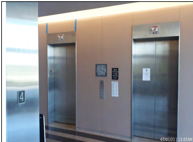
Van Nuys Courthouse West Elevator Replacement - After
