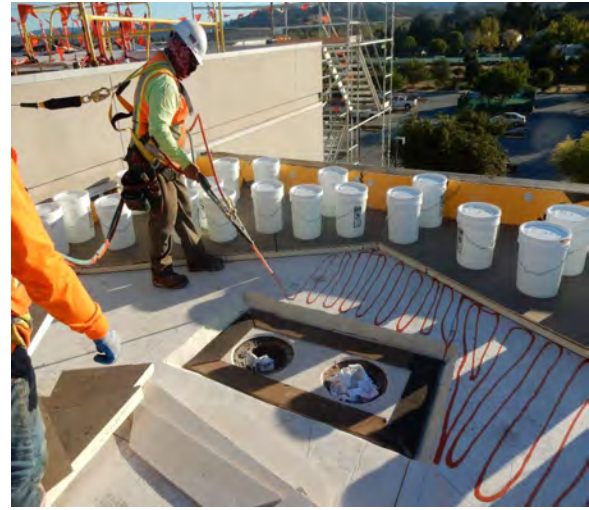
Morgan Hill Courthouse – Roof
