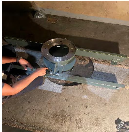
Harbor Justice Center-Newport Beach - Elevators
