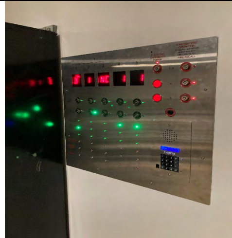
El Monte Courthouse Elevator Replacement
