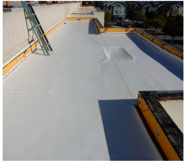
Morgan Hill Courthouse – Roof
