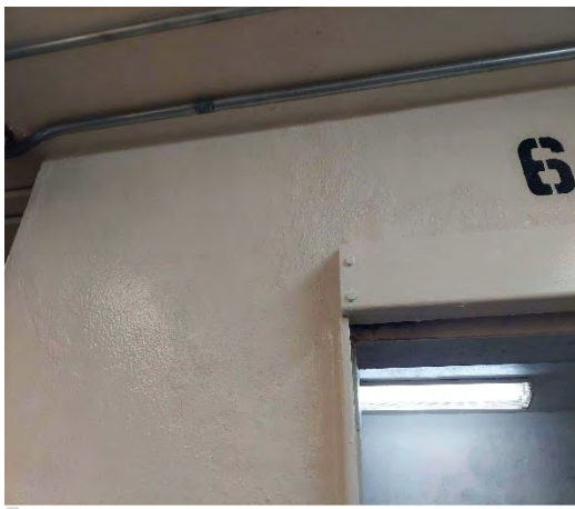
Newly repaired/painted wall
