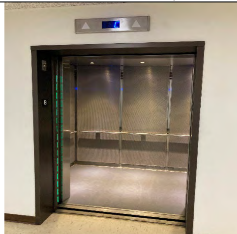
El Monte Courthouse Elevator Replacement
