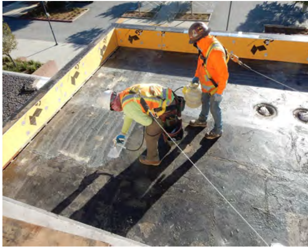
Morgan Hill Courthouse – Roof
