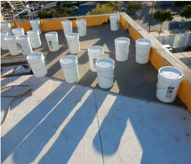
Morgan Hill Courthouse – Roof
