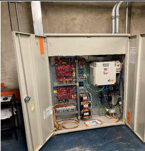
El Monte Courthouse Elevator Replacement
