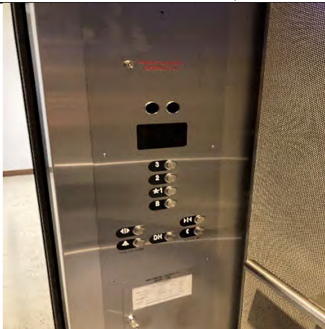
El Monte Courthouse Elevator Replacement
