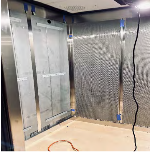
Harbor Justice Center-Newport Beach - Elevators
