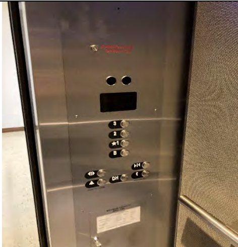
El Monte Courthouse Elevator Replacement
