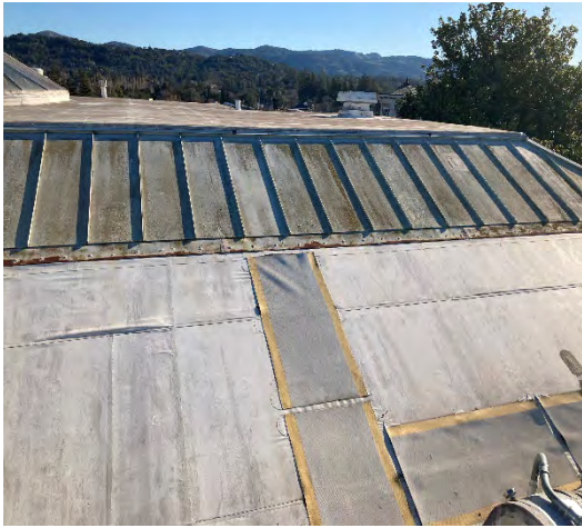
Historic Courthouse – Roof
