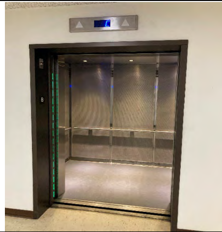
El Monte Courthouse Elevator Replacement
