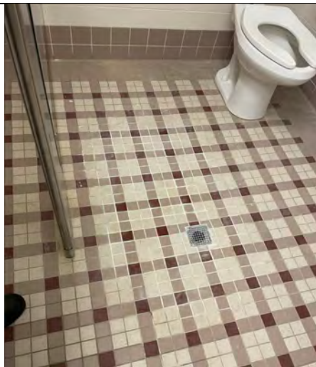
Newly repaired floor drain
