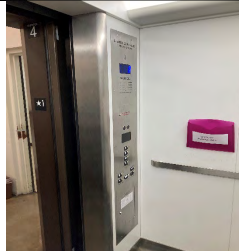
El Monte Courthouse Elevator Replacement
