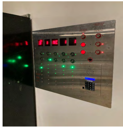
El Monte Courthouse Elevator Replacement
