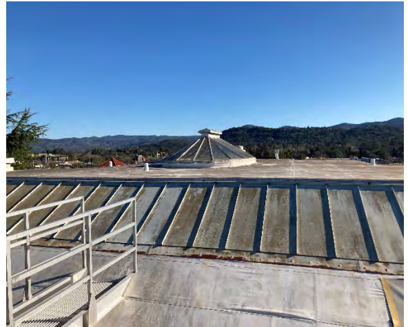
Historic Courthouse – Roof
