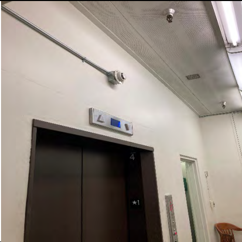
El Monte Courthouse Elevator Replacement
