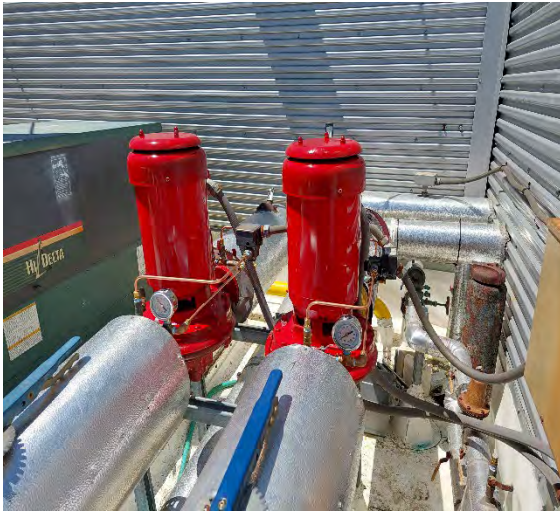
Criminal Court Building - BMS
