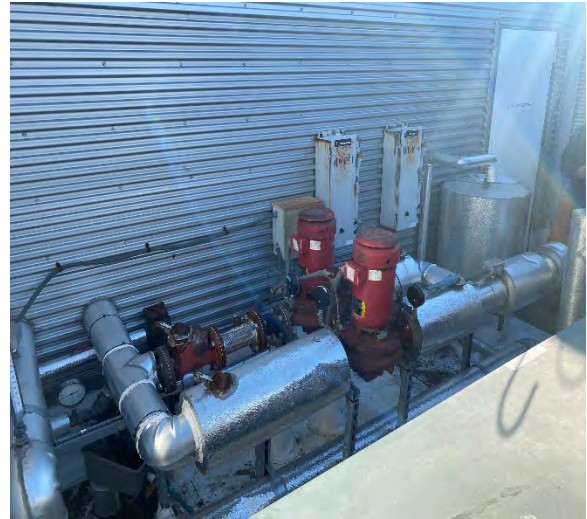
Criminal Court Building - BMS
