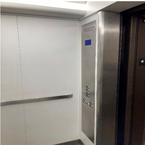
El Monte Courthouse Elevator Replacement
