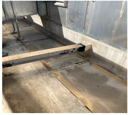
Historic Courthouse – Roof
