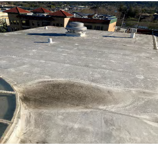
Historic Courthouse – Roof
