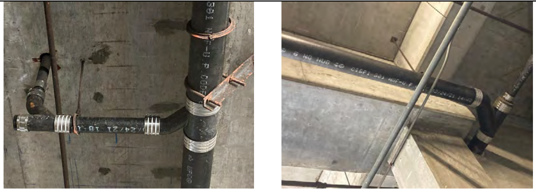
Newly replaced drain pipes and drain lines
