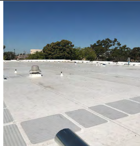
Torrance Annex Roof Replacement
