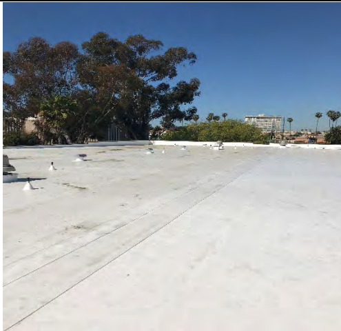
Torrance Annex Roof Replacement
