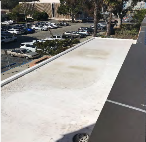
Torrance Annex Roof Replacement
