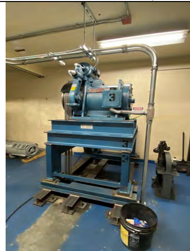
El Monte Courthouse Elevator Replacement
