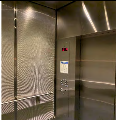
Edmund D. Edelman Elevator Replacement
