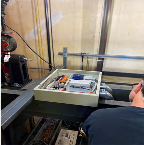
El Monte Courthouse Elevator Replacement
