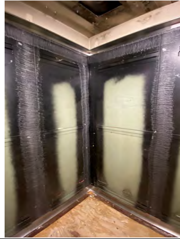
El Monte Courthouse Elevator Replacement
