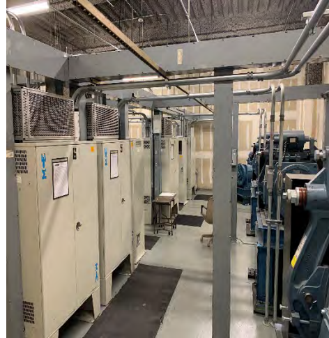
Edmund D. Edelman Elevator Replacement
