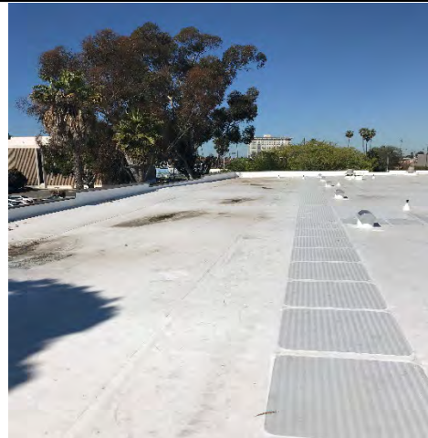
Torrance Annex Roof Replacement
