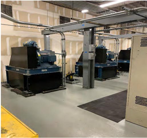
Edmund D. Edelman Elevator Replacement
