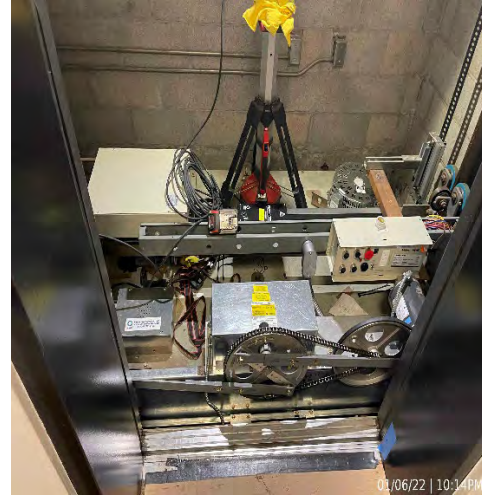
Fremont Hall of Justice Elevator Replacement
