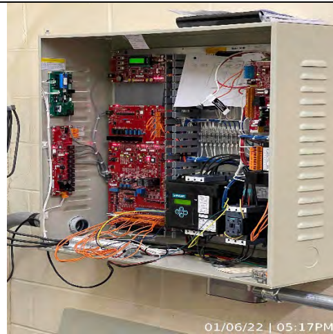
Fremont Hall of Justice Elevator Replacement
