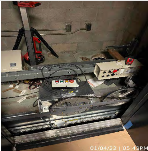
Fremont Hall of Justice Elevator Replacement
