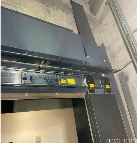
Fremont Hall of Justice Elevator Replacement
