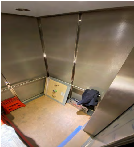
El Monte Courthouse Elevator Replacement
