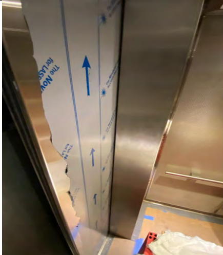
El Monte Courthouse Elevator Replacement
