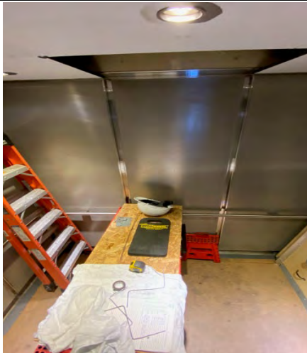
El Monte Courthouse Elevator Replacement
