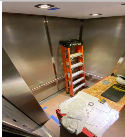
El Monte Courthouse Elevator Replacement
