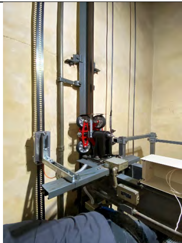
El Monte Courthouse Elevator Modernization
