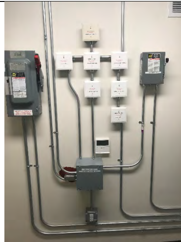
Northern Branch Courthouse Elevator Modernization
