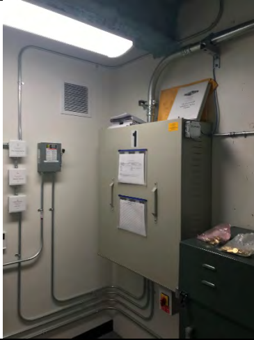
Northern Branch Courthouse Elevator Modernization
