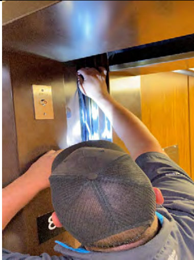
El Monte Courthouse Elevator Modernization
