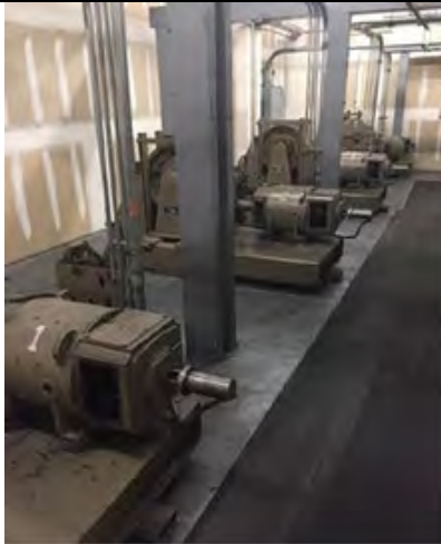
Edelman Children's Court Elevator Modernization
