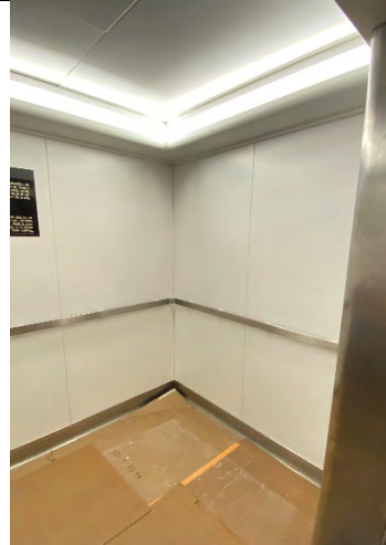
El Monte Courthouse Elevator Modernization
