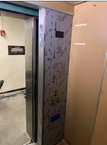
NCRC Elevator Modernization
