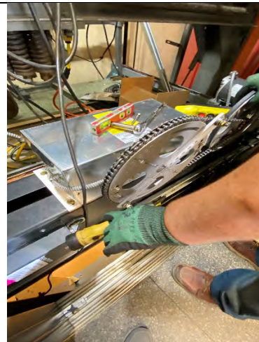
El Monte Courthouse Elevator Modernization
