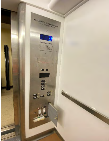
El Monte Courthouse Elevator Modernization
