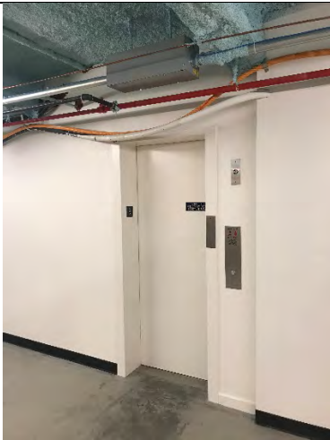
Northern Branch Courthouse Elevator Modernization
