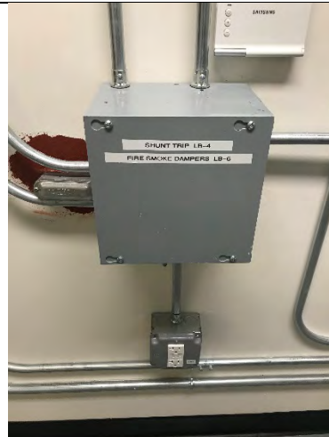
Northern Branch Courthouse Elevator Modernization
