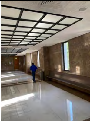
Pomona Courthouse South – Fire Protection
