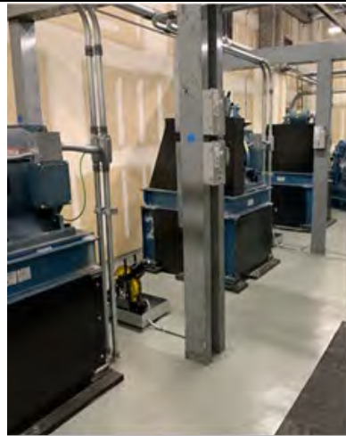
Edelman Children's Court Elevator Modernization
