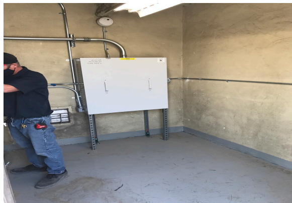
Barstow Courthouse – San Bernardino – Elevator
