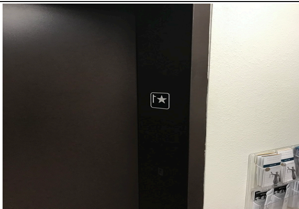
Barstow Courthouse – San Bernardino – Elevator
