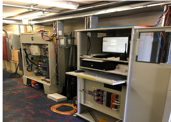
Torrance Courthouse – LA – Elevator
