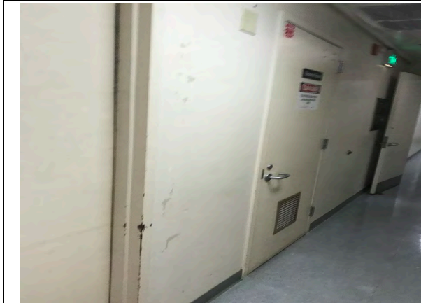
Burbank Courthouse – LA – Elevator
