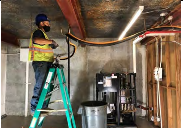
Northern Branch Courthouse – San Mateo – Elevator
