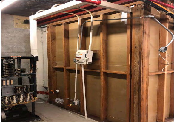
Northern Branch Courthouse – San Mateo – Elevator
