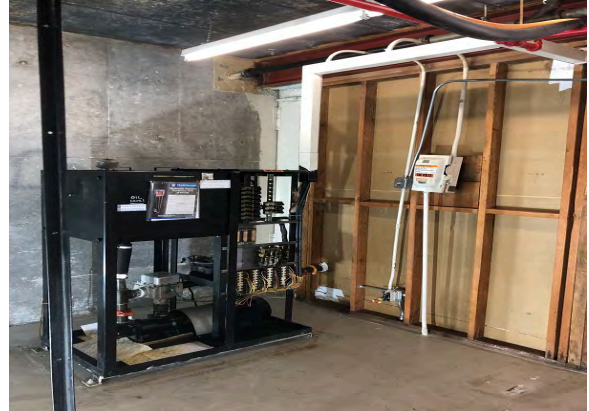
Northern Branch Courthouse – San Mateo – Elevator
