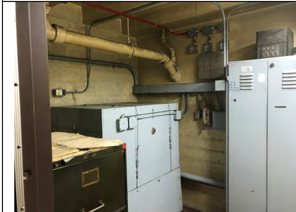
Burbank Courthouse – LA – Elevator
