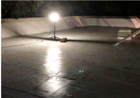
Santa Clara Courthouse - Santa Clara - Roof
