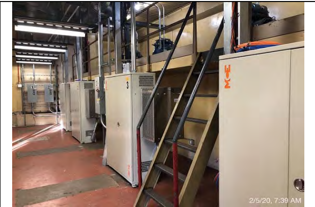
Inglewood Courthouse - LA - Elevator
