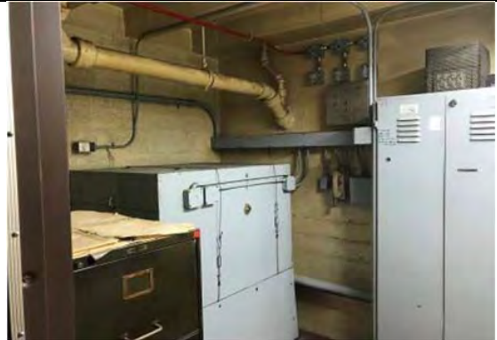
Burbank Courthouse - LA - Elevator
