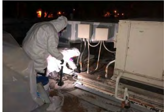
Santa Clara Courthouse - Santa Clara - Roof
