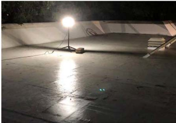
Santa Clara Courthouse - Santa Clara - Roof
