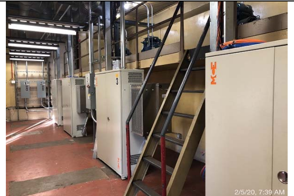
Inglewood Courthouse - LA - Elevator
