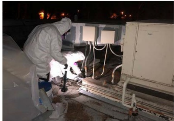
Santa Clara Courthouse - Santa Clara - Roof
