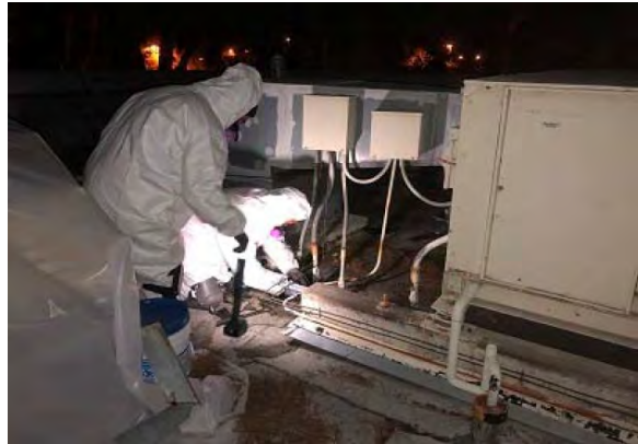
Santa Clara Courthouse - Santa Clara - Roof
