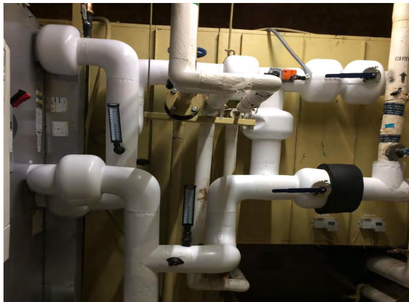
Newly replaced water control valves
