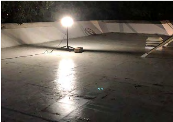
Santa Clara Courthouse - Santa Clara - Roof
