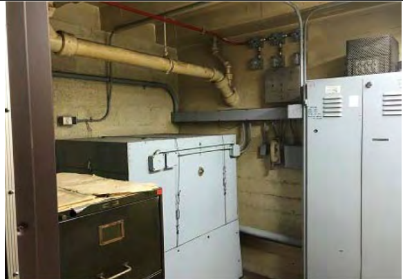
Burbank Courthouse - LA - Elevator
