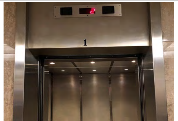
Inglewood Courthouse - LA - Elevator
