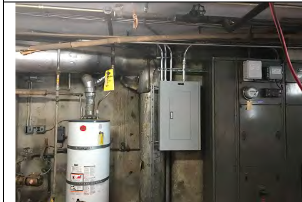
Inglewood Juvenile Courthouse - LA - Elevator
