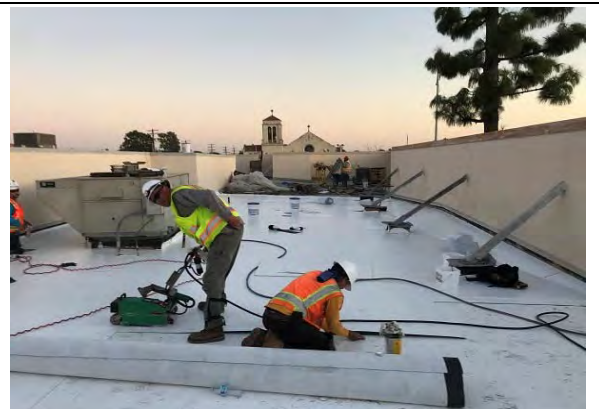
Delano Courthouse - Kern - Roof
