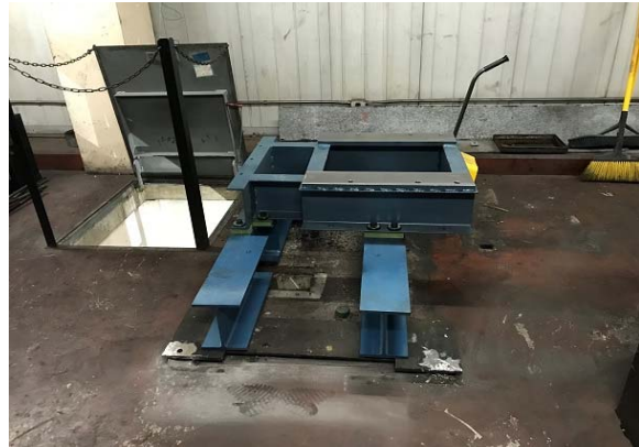
Inglewood Courthouse – LA - Elevator
