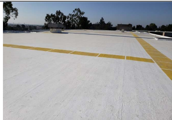
North Justice Center – Orange - Roof
