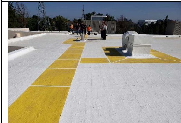
North Justice Center – Orange - Roof
