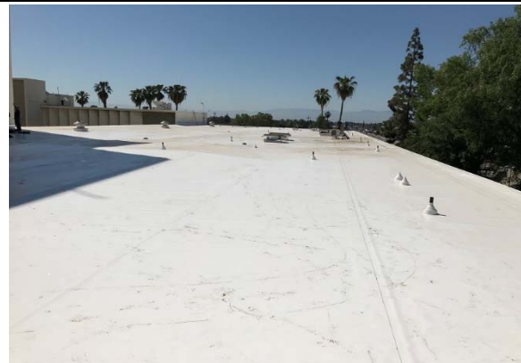
Bakersfield Superior Court - Kern - Roof
