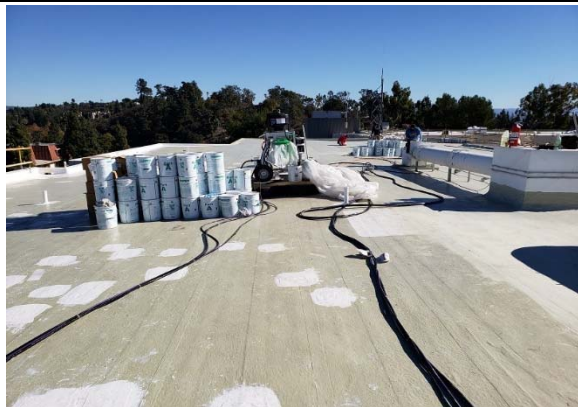
North Justice Center - Fullerton - Roof
