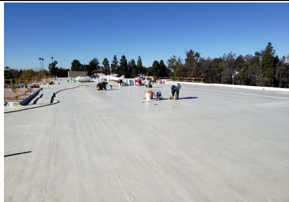
North Justice Center - Fullerton - Roof
