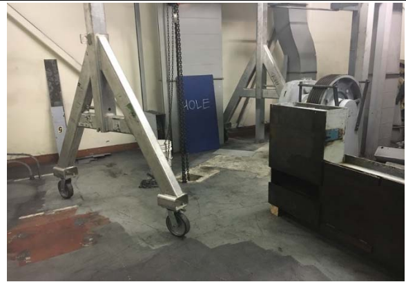
Alhambra Courthouse - LA - Elevator
