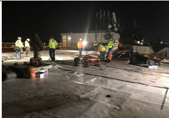
Bakersfield Superior Court - Kern - Roof
