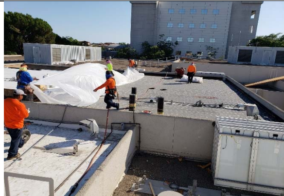
North County Regional Center - San Diego - Roof
