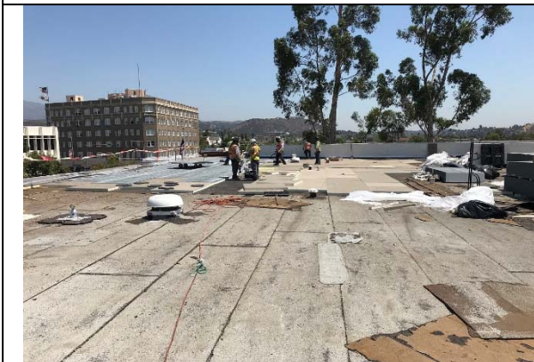
Glendale Courthouse - Glendale - Roof
