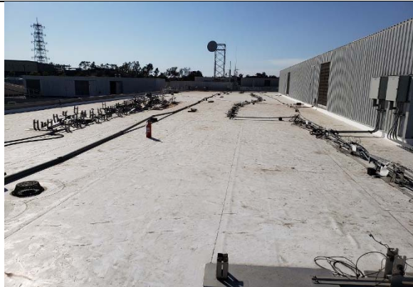
North County Regional Center - San Diego - Roof
