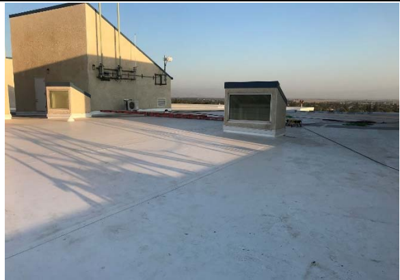
Bakersfield Juvenile Center – Bakersfield - Roof
