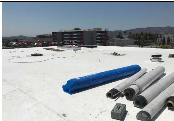
Glendale Courthouse - Glendale - Roof
