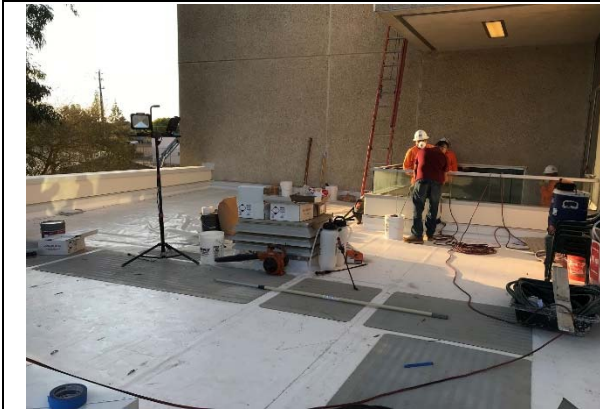
Bakersfield Juvenile Center – Bakersfield - Roof
