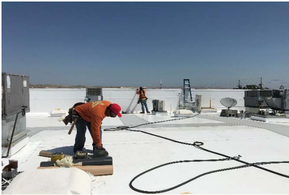
Taft Courthouse - Taft - Roof
