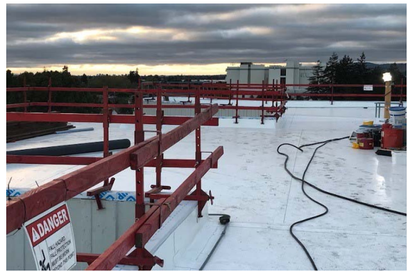
Hall of Justice - Hayward - Roof
