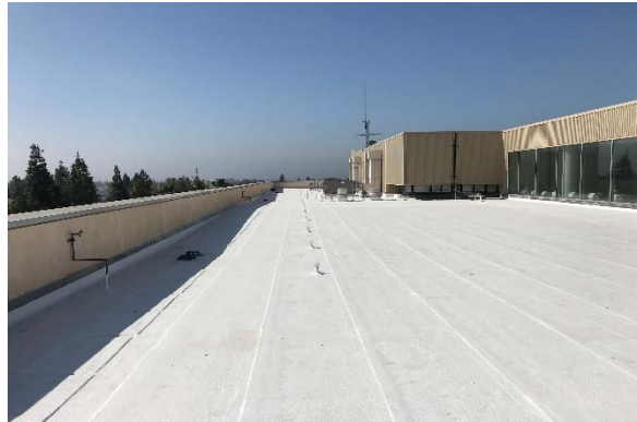
Chatsworth Courthouse - Chatsworth - Roof
