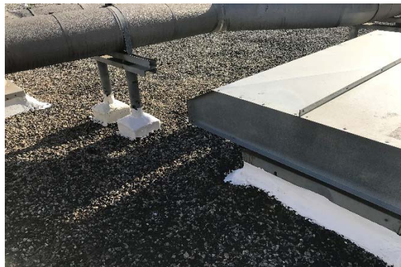
East Los Angeles Courthouse - L.A. - Roof
