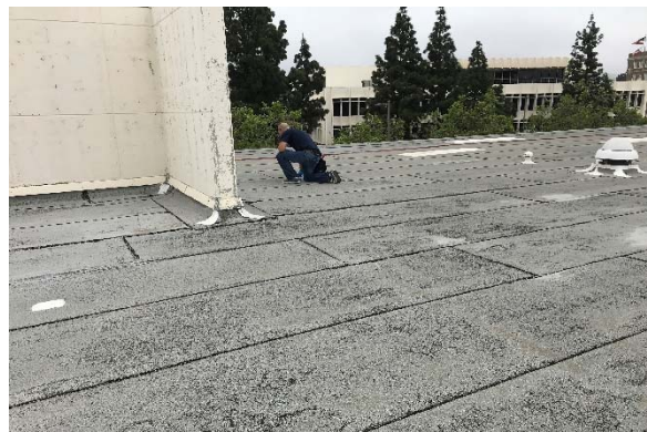
Glendale Courthouse - Glendale - Roof
