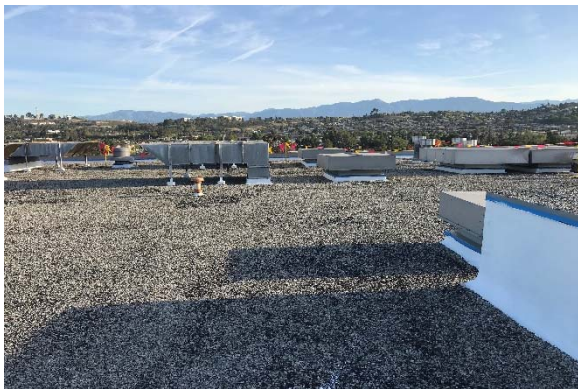
East Los Angeles Courthouse - L.A. - Roof
