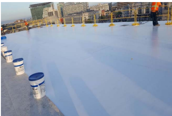
Civic Center Courthouse - San Francisco - Roof
