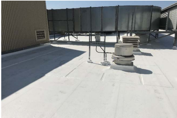
Chatsworth Courthouse - Chatsworth - Roof
