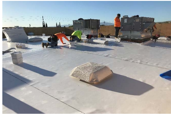
Taft Courthouse - Taft - Roof
