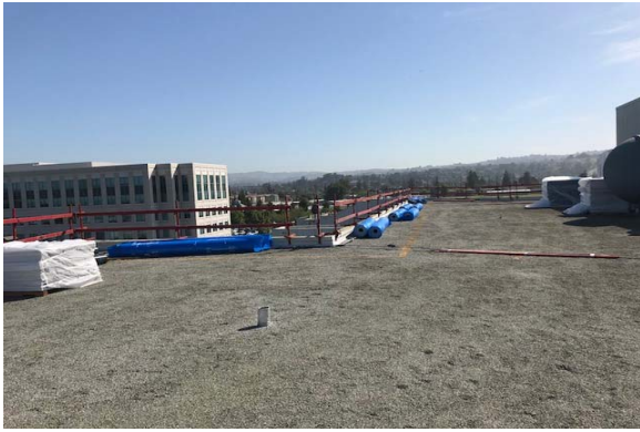
Hall of Justice - Hayward - Roof
