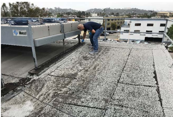
Glendale Courthouse - Glendale - Roof
