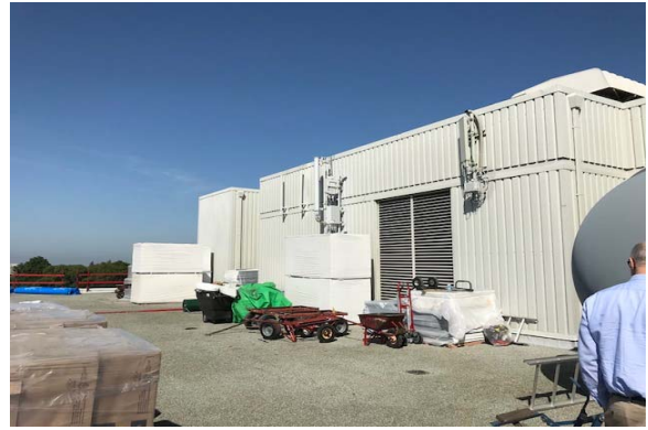
Hall of Justice - Hayward - Roof
