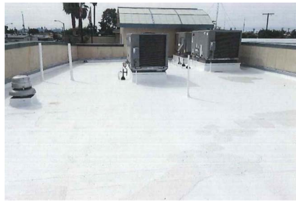
Blythe Courthouse- Superior Court Roof
