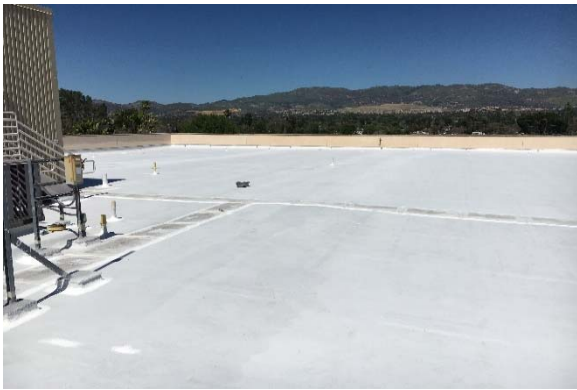
Chatsworth Courthouse Roof
