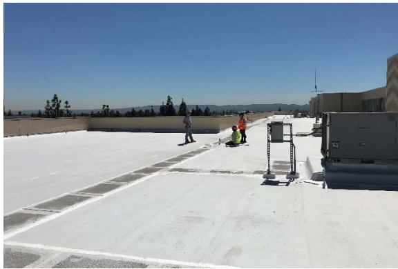
Chatsworth Courthouse Roof
