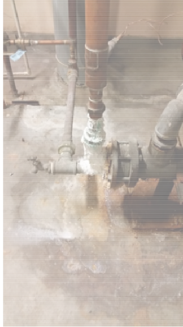
Above: Existing, failing valves and pump Below: Newly replaced valves and pump
