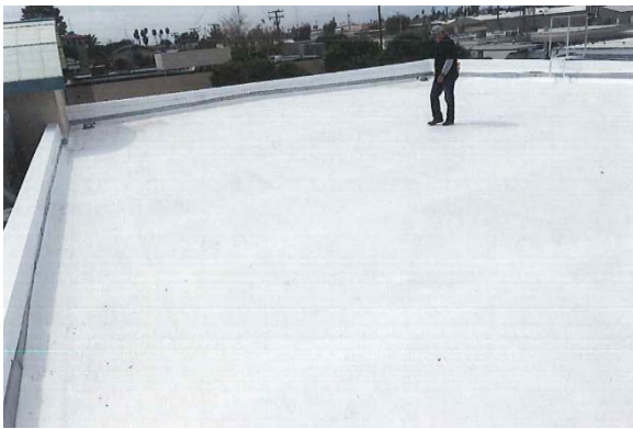
Blythe Courthouse – Superior Court Roof
