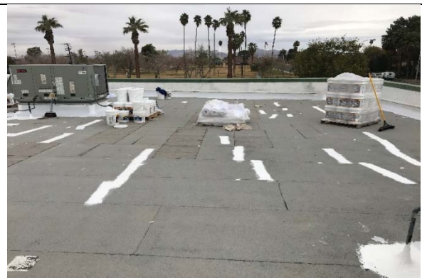
Blythe Courthouse- Superior Court Roof
