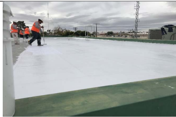
Blythe Courthouse – Superior Court Roof
