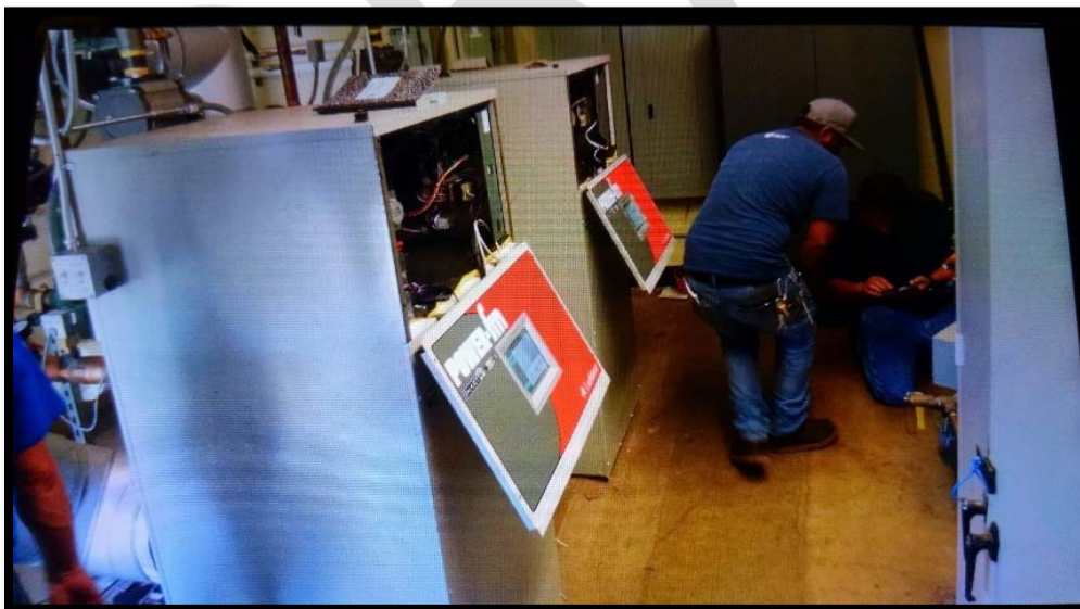
Above: Failing existing 3 MBTU Boiler (Parts no longer being fabricated). Below: New 1.4 BTU Boilers (No operating permits required and much more efficient).
