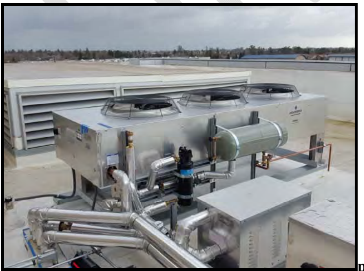
Below: Tuning up by making final adjustments to the units Right: New roof top condensing unit.
