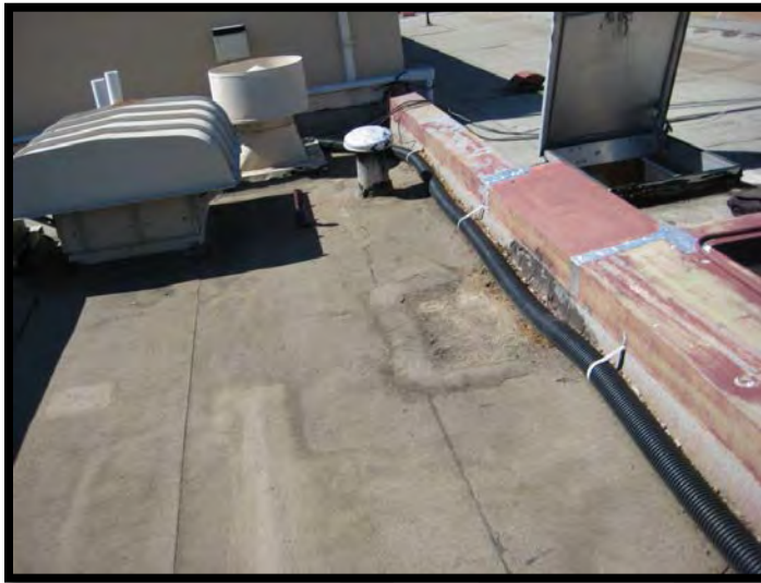
Before: The old roof, showing bubbles and delaminating, where water intrusion occurs ( above ). After: The new, energy efficient roof ( right ).
