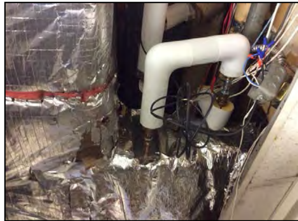
Above Left: Before – Rusted and leaking units. Above Right: After – Clean and insulated units.
