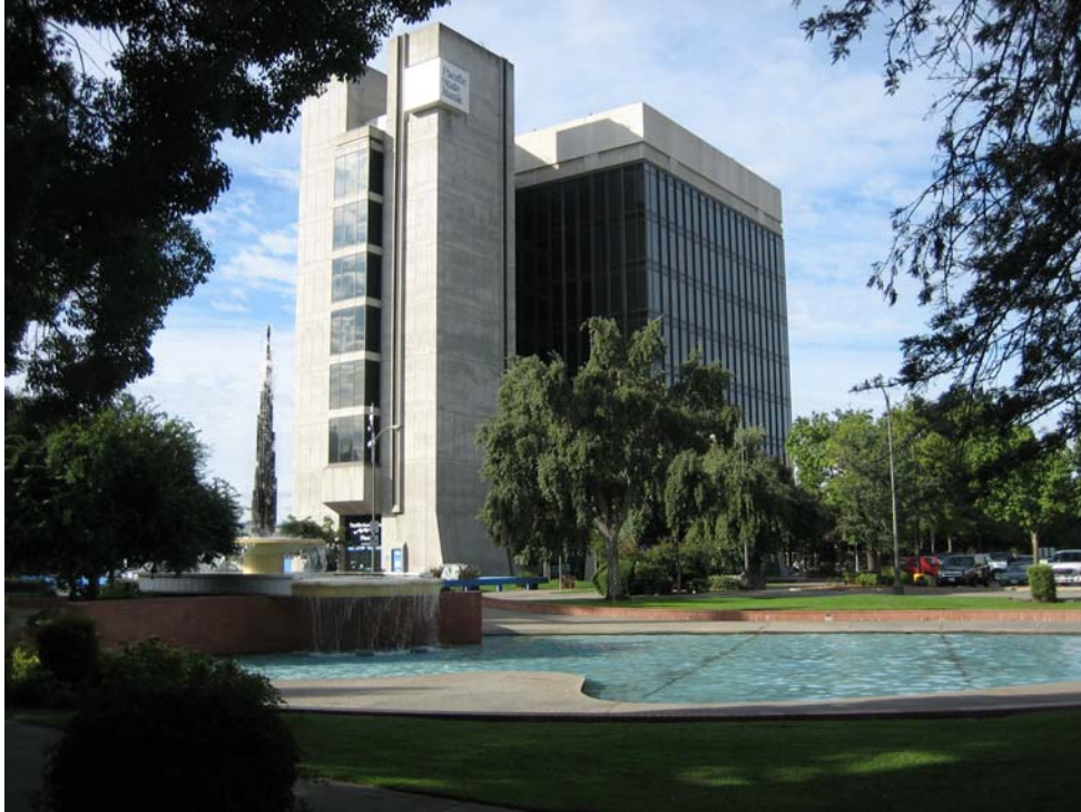
Figure C7. View Southwest From Courthouse Sidewalk Near West Entrance
