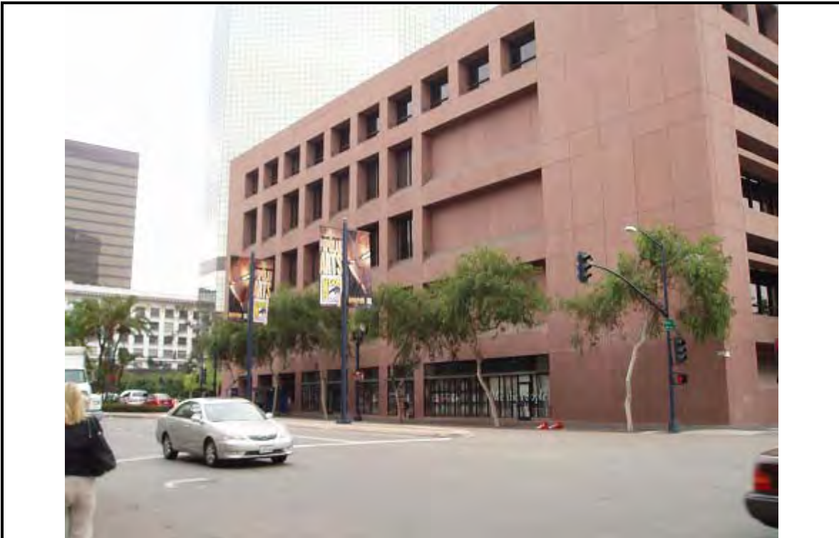
PHOTOGRAPH 1 DESCRIPTION: Federal Courthouse located Southeast of Subject Property Date: 10 July 2007 ERM 330 West Broadway San Diego, CA
