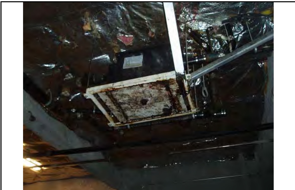
PHOTOGRAPH 10 | DESCRIPTION: Parking Garage Level One - Grease Trap for Food Court
