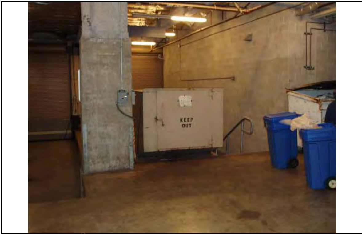
PHOTOGRAPH 13 | DESCRIPTION: Loading Dock - Compactor
