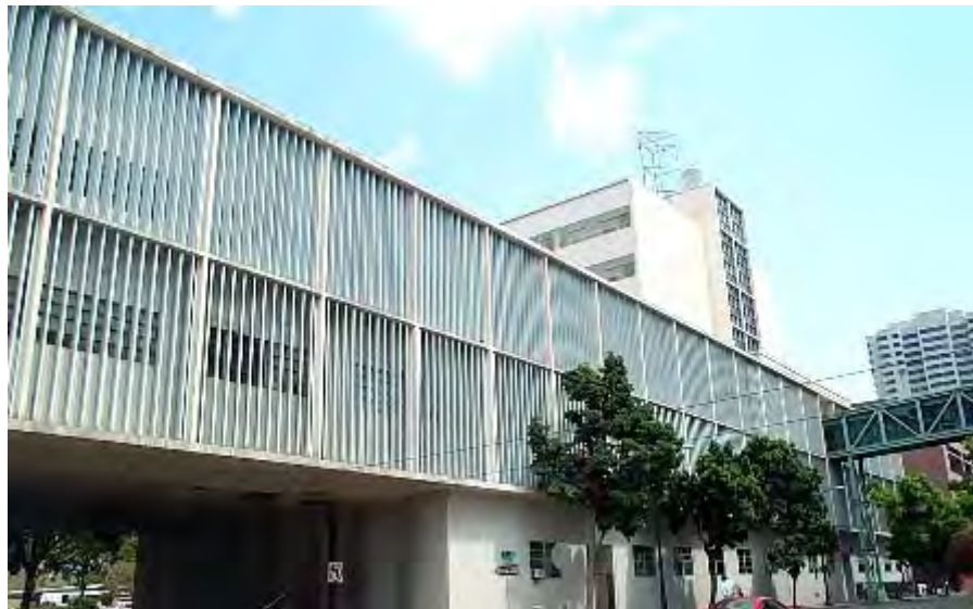
West Elevation at C Street Bridge (37-A1-E, 37-A1-A)
