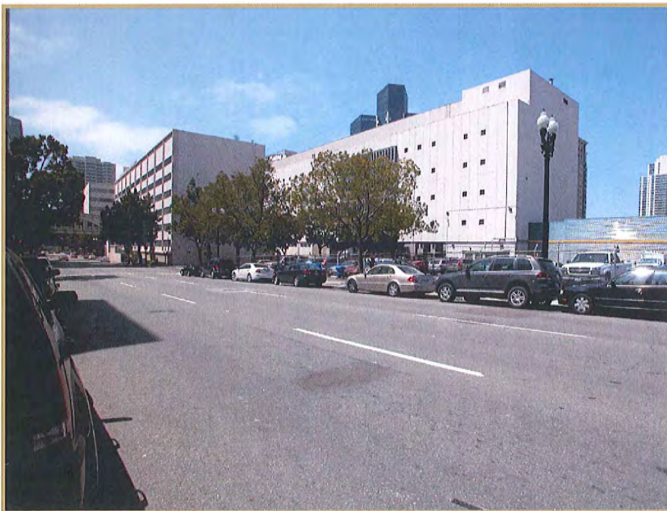
Plate 4: View of Detention Center, taken from east side of Front Street, facing south-southeast
