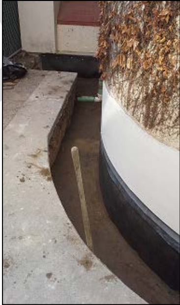
Above: the faulty membrane on the exterior of the building as it looked at time of failure (with dirt excavated). Near Right: Repair effort on the membrane. Far Right: The restored men’s restroom.
