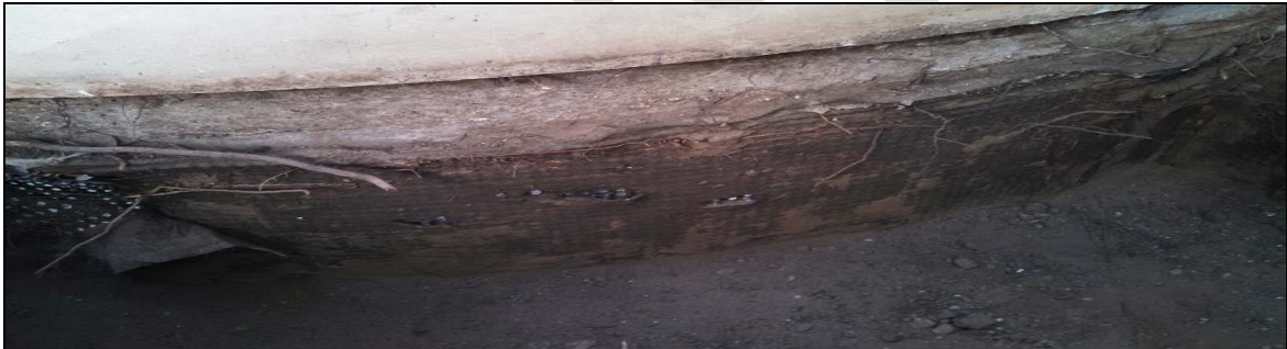
Above: the faulty membrane on the exterior of the building as it looked at time of failure (with dirt excavated). Near Right: Repair effort on the membrane. Far Right: The restored men’s restroom.
