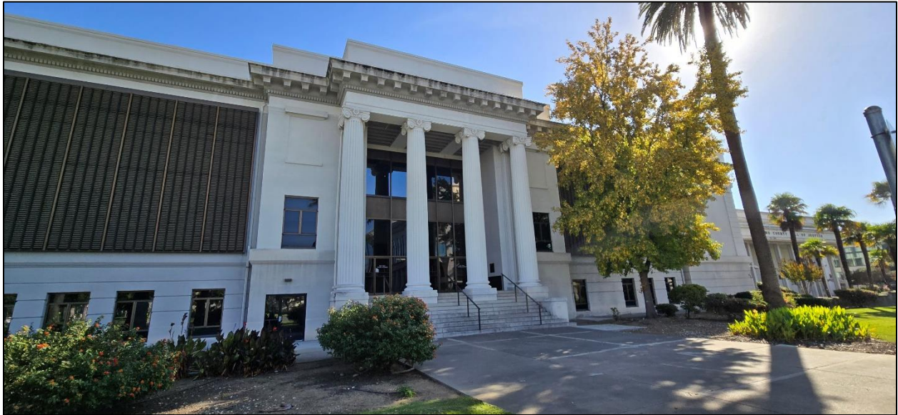
Photo 1. Existing Hall of Justice Building (North Wing) at 600 Union Avenue.
