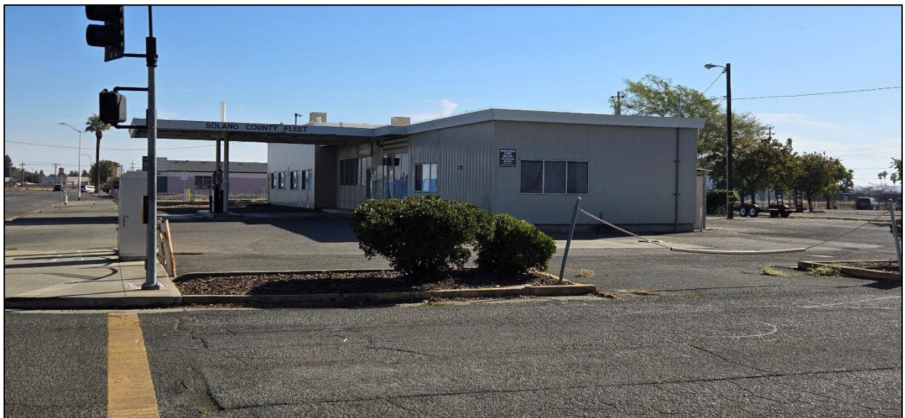
Photo 10. Existing Solano County Fleet building at 447 Texas Street, east of the project site.
