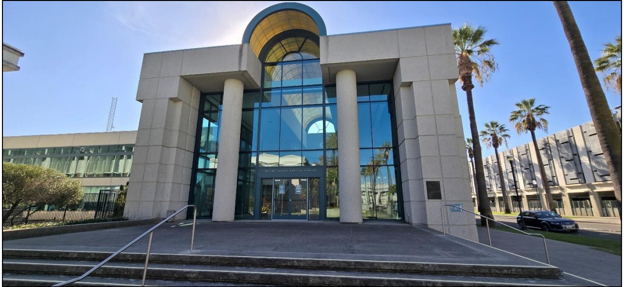
Photo 7. Existing Solano County Justice Center building at 500 Union Avenue, west of the project site.
