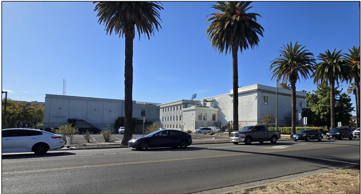
Photo 6. Viewing south toward the project site from the north side of Texas Street.
