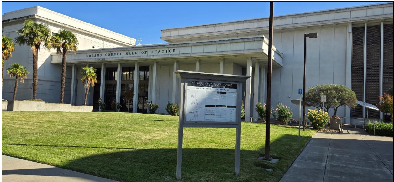
Photo 2. Existing Hall of Justice (South Wing) at 550 Union Avenue.
