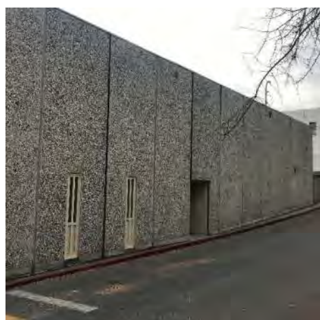
Figure 17. Annex, north façade, view southwest (ARG, 2022)
