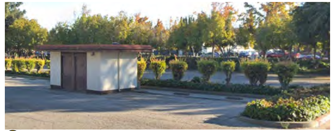
7. Site structure to be demolished and resurfaced for parking.
