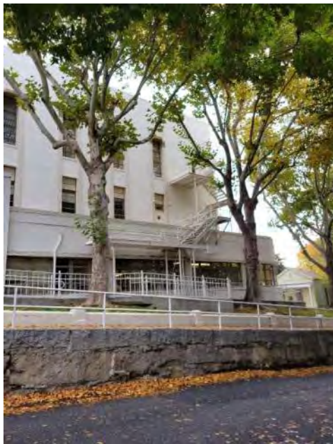
Figure 6. Granite retaining wall and low concrete wall at west side of the site, view east (ARG, 2022)
