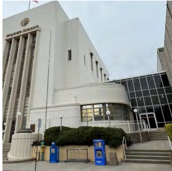
Figure 11. Primary (south) and east façades, view northwest, showing 1937-constructed elements including curved first-floor volumes and entry details, and 1964-constructed connecting corridor to the Annex (at right) (ARG, 2022)
