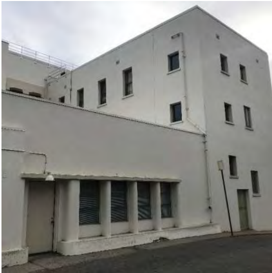
Figure 10. North (rear) façade, view southwest, showing the 1937-constructed sheriff's office at left and pre-1937 jail at right, with 1937 alterations (extent of alterations unknown) (ARG, 2022)
