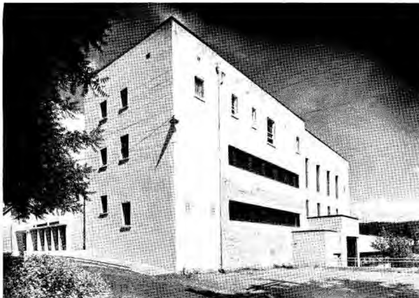
View from northwest showing jail section
