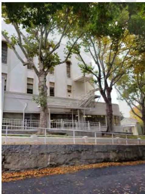
Figure 6. Granite retaining wall and low concrete wall at west side of the site, view east (ARG, 2022)
