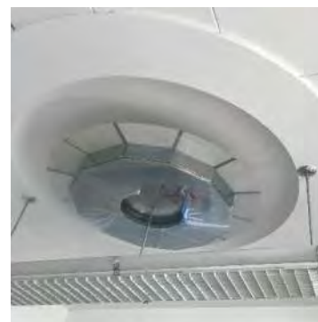
Figure 14. Recessed circular light fixture (ARG, 2022)
