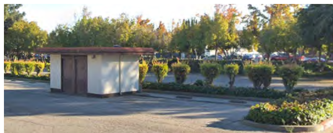
7. Site structure to be demolished and resurfaced for parking.
