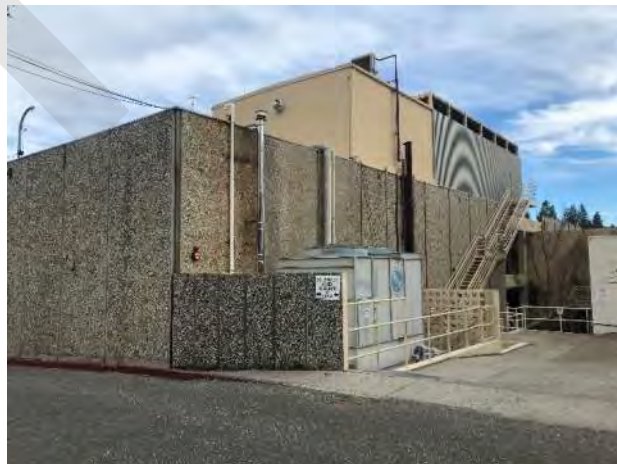
Figure 18. Annex, west façade, north portion, showing HVAC, penthouse, and exterior egress, view southeast (ARG, 2022)
