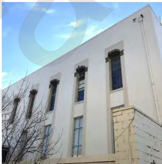
Figure 9. East façade, view southwest, showing fenestration pattern and material, including replacement second-floor windows and CMU enclosure (ARG, 2022)
