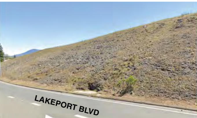
fig. 2.1 Courthouse site on bench 50' above Lakeport Blvd.
