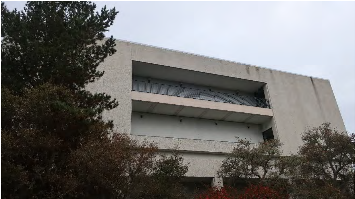
Photo 2: Courthouse Building East Elevation
