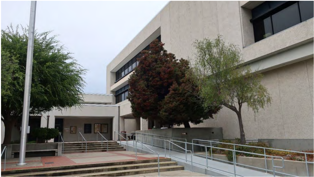
Photo 1: Courthouse Building Entrance
