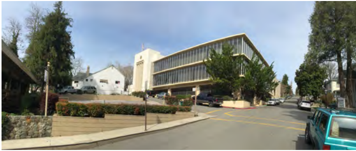
View of Annex
