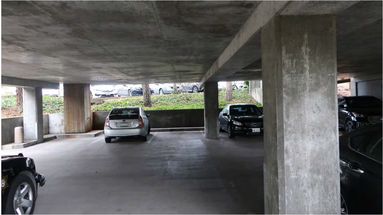
Photo 4: Parking Garage Interior
