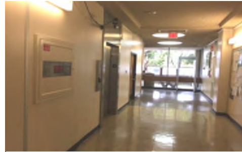
Figure 1 - Fire Hose inside the B Level public hallway
