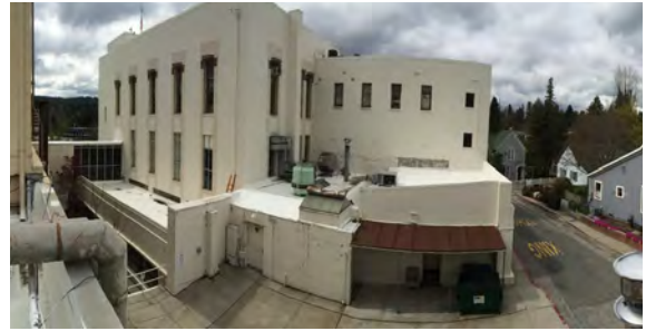
Historic Courthouse Wing, and relationship to context
