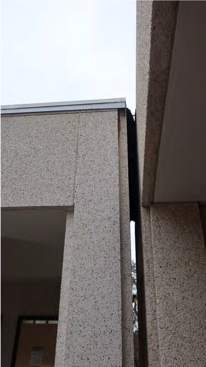
Photo 3: Seismic Gap Between Courthouse and Annex
