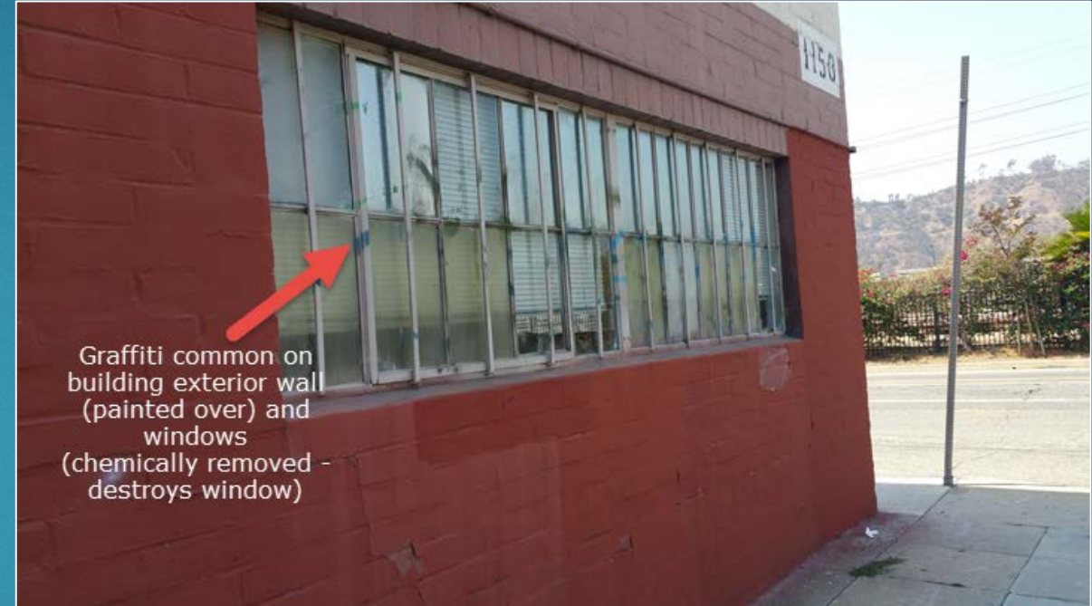
Exterior wall with residual graffiti and damaged windows
