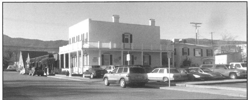
Eddy Street Annex is non-compliant with ADA & has no security
