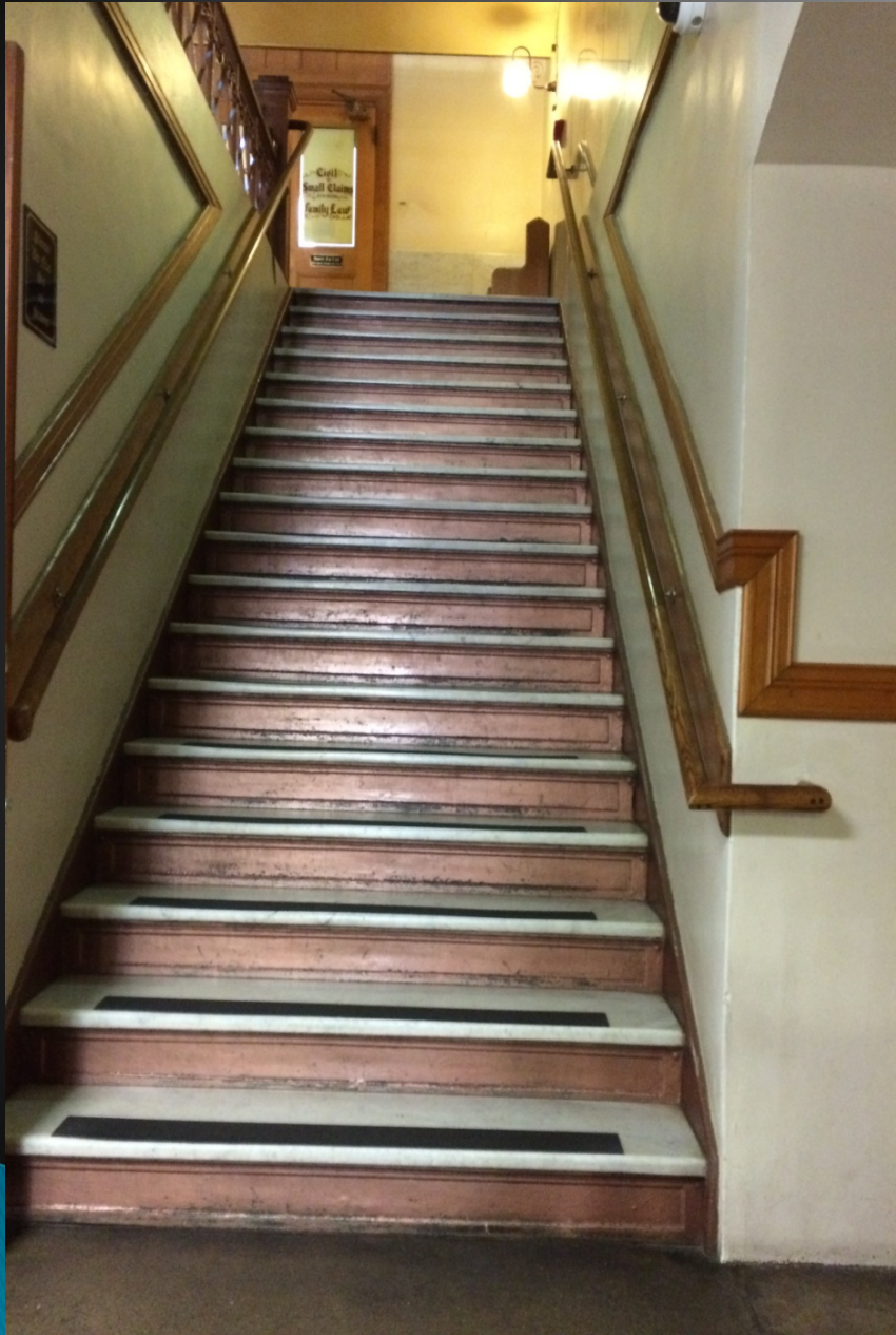
View of stairs from first to second floor.
