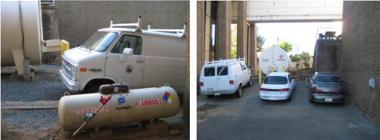
Photos of the two fuel tanks located between the courthouse on the left and the old jail on the right.
