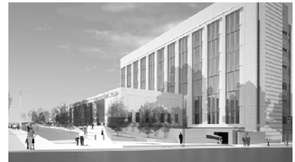
View looking Northeast
