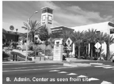
B. Admin. Center as seen from site
