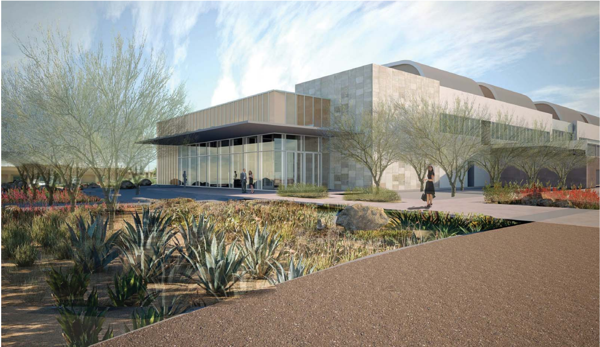
VIEW FROM PARKING LOT TOWARD ENTRY
