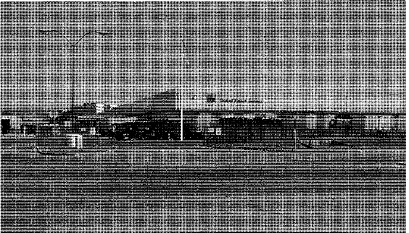
2b - UPS Shipping/Distribution Center
